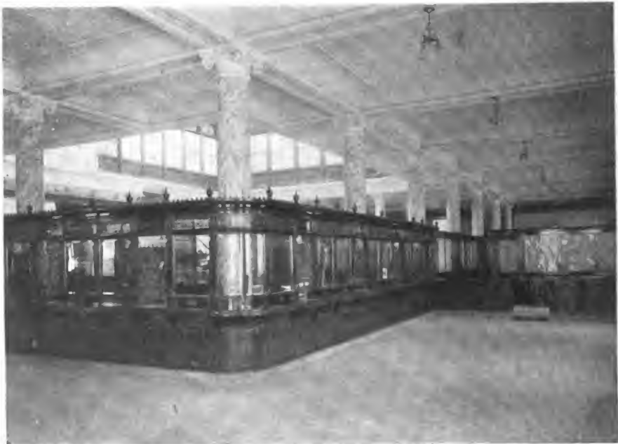
Main Banking Room BANCO CENTRAL MEXICANO.
